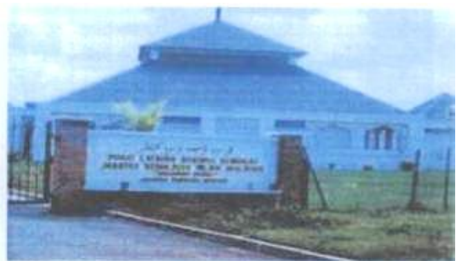
Construction of Pusat Latihan Dakwah Keningau, Sabah (1997)
